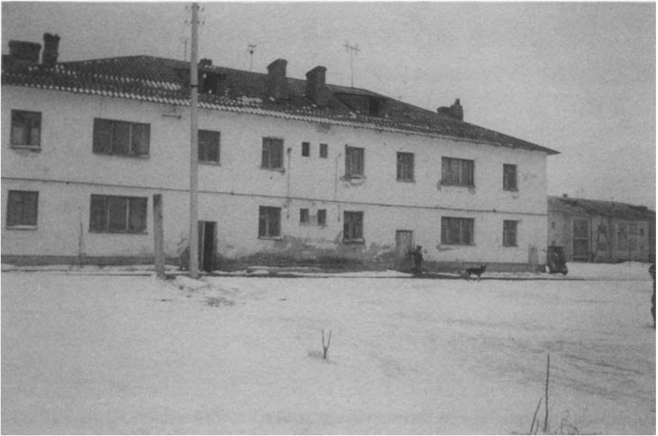
Figure 14.2 At Verchnyua Troitsa , one of the new village's two-storey houses, each containing 16 flats
